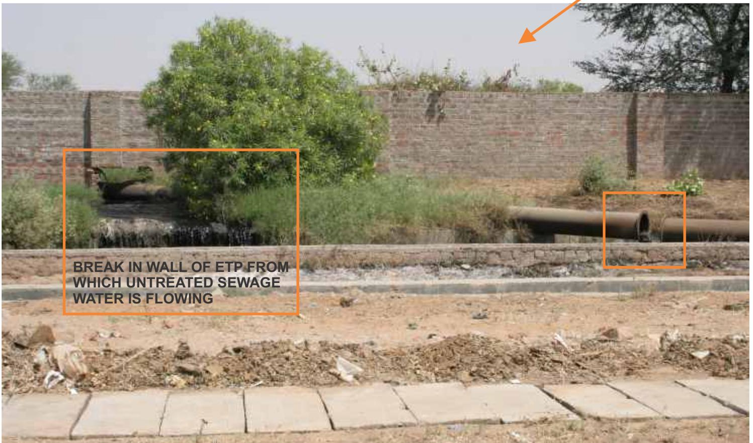
**BREAK IN WALL OF ETP FROM WHICH UNREATED SEWAGE WATER IS FLOWING**
