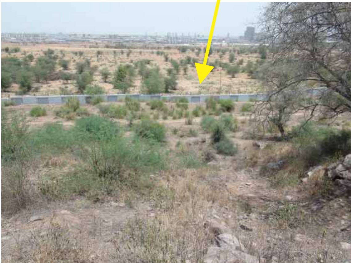
View of the maruti land from the top of the hill near the school, the wall is blocking the water flow system that existed here for centuries.
